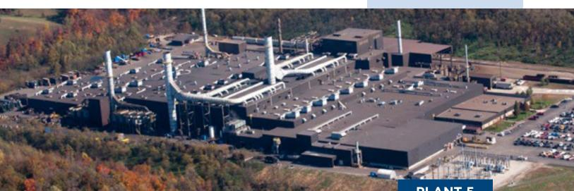
Iron Type: Gray iron, ductile iron, and compacted graphite Melt capacity: 160 tons per hour Markets served: Light vehicle, commercial vehicle, agriculture, and construction Products manufactured: Brake rotors and drums, brake calipers, crankshafts, differential carriers, differential cases, and flywheel housings
