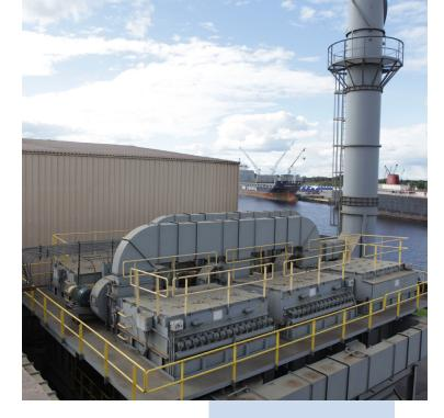
control systems at each plant. In most cases, this technology is not mandated by a regulatory agency but utilized as an elective continuous improvement. Because even small holes can affect the performance of baghouse filters, these probes are used to monitor the integrity of the baghouses and performance of the filtration system.
